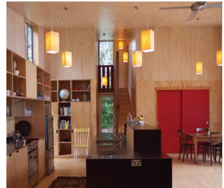
To keep waste and costs to a minimum, the interior of the house was built in natural pine plywood throughout, limewashed above 2.4 metres for effect. opposite page The building's footprint was shaped to incorporate the mature trees surrounding it, in order to connect with the existing natural environment.
